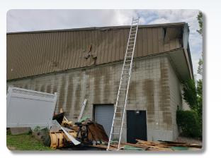
to The Cove at Yarmouth on the other side of Mill Creek, formerly known as the Howard Johnson Motel). The debris from the Cape Sands' roof was blown over the creek slamming into the gable end of the RSC building. Approximately one third of the corrugated sheet metal wall was dented and torn open on the end. Twenty plus vehicles experienced some sort of windshield and/or body damage as the debris was scattered throughout the 500-parking lot area.
